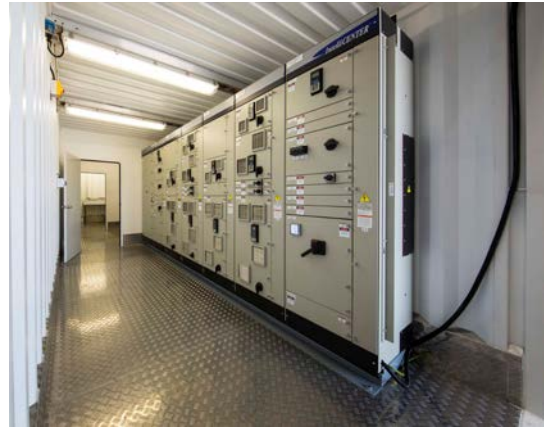
The MCC features the complete Rockwell Automation Connected Components range, including E300 Electronic Overloads and PowerFlex 525 and 753 drives all on an Ethernet backbone.
