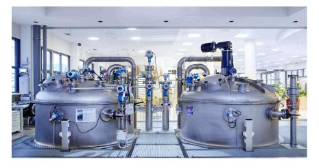
The oil tank facility is located on two levels. It consists of two tanks with a capacity of 24,000 liters. Another tank with a capacity of 1,600 liters facilitates filling a main tank up to the lid.
